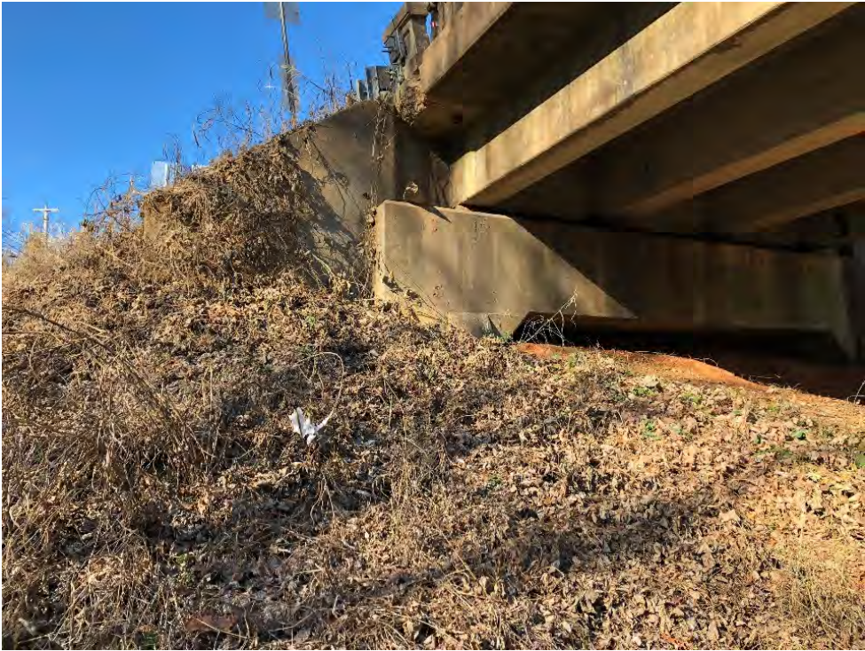
Super/Sub Structure – Abutment 1
