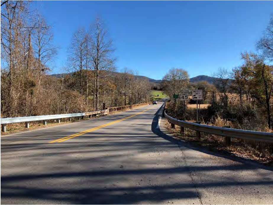
Eastbound Bridge Approach
