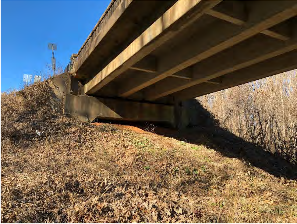
Super/Sub Structure – Abutment 1
